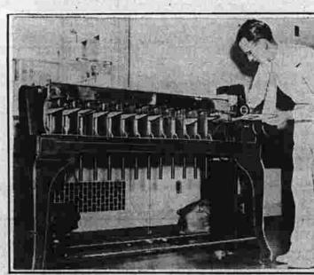
This superhuman machine sorts and identifies finger-prints automati-cally. Varying perforations on the finger-print record cards, according pictures and other data on the wanted man or men. These to the type, cause the cards to drop into stacks as they pass through the are widely distributed, going all over the country by airmail, machine. Within two minutes, almost any given print can be found. in some cases more than a million copies,
